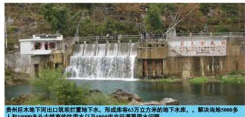
贵州巨木地下河出口筑坝拦蓄地下水，形成库容63万立方米的地下水库，解决当地5000多人和10000多头大牲畜的饮用水以及6000亩农田灌溉用水问题。 A dam was built up at the outlet of Jumu Underground River, Guizhou, China, which has generated a reservoir with the capacity of 630,000 m 3 . The water level was enhanced by 20m, and a hydropower station was established. More than 5,000 local people and over 10,000 large livestock lived on this reservoir, as well as 6,000 mu farmlands were irrigated by this reservoir. (1 mu=0.067 ha)
