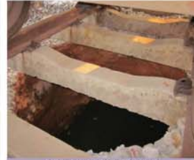
岩溶塌陷对油气管道工程的影响 The harm of karst collapse to oil and gas pipelines
